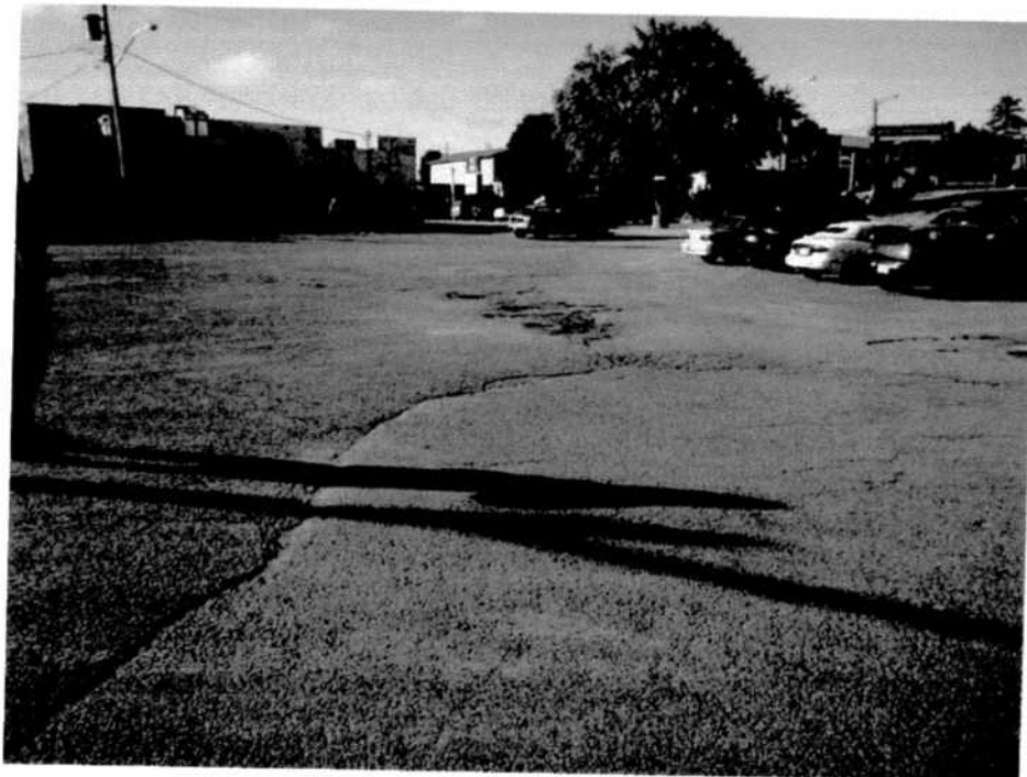
Photograph 2. Asphalt Over Culvert ↑
