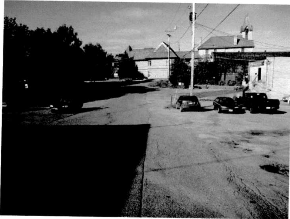
Photograph 1. Looking West at Roadway over Culvert ↑
