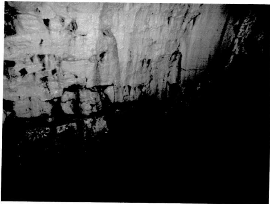
Photograph 6. Encrustation of Barrel ↑
