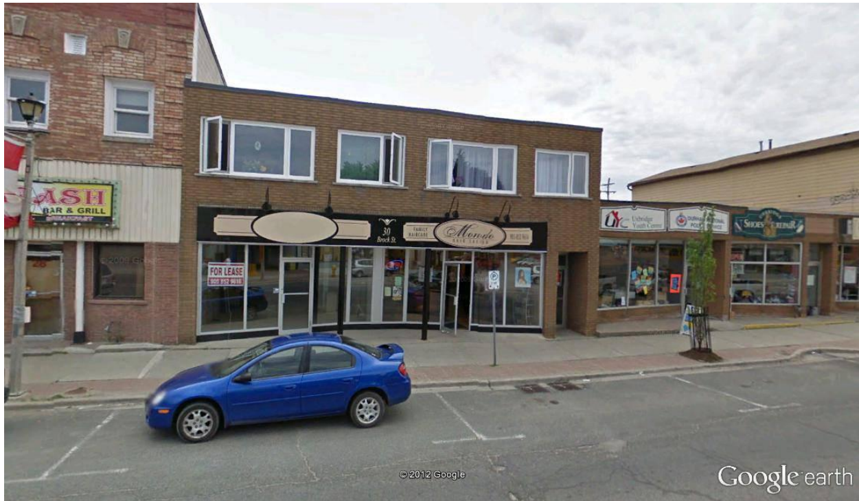
Image 5: Looking south along Brock Street at existing buildings to be impacted by culvert replacement. (Google, 2009)
