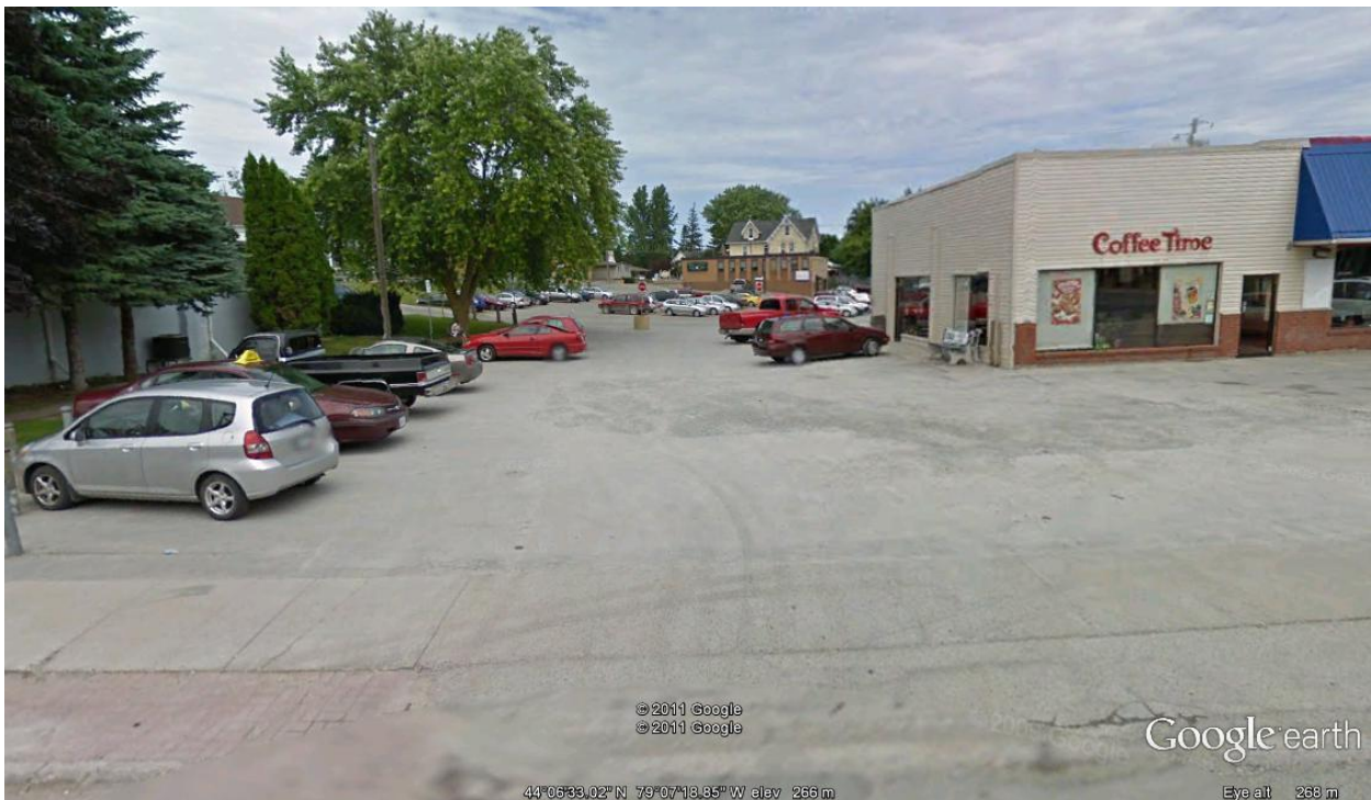
Image 4: Looking northwest along Brock Street at existing paved area to be impacted by culvert replacement. (Google, 2009)
