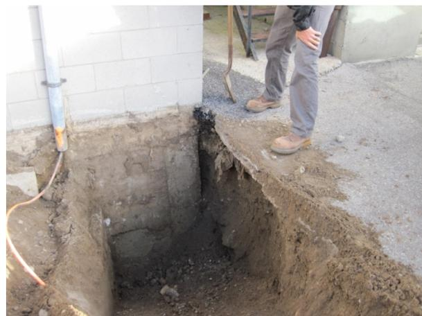
**Figure 6. Exposure of building foundation at #34 Brock Street**
